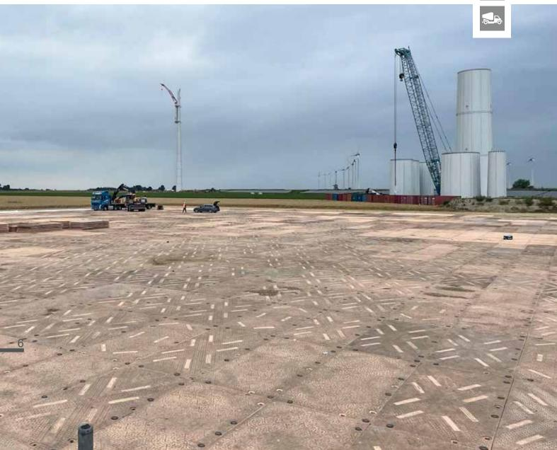
Engineered for performance and strength, the interlocking overlap mats distribute weight across a large surface area while remaining stable and strong through all operating conditions. The IsotractionTM surface tread improves traction and safety for load-bearing vehicles, while the patented Four3 connection system reduces mat drift and slippage. The mats provide years of reusable performance with proper use and maintenance.
